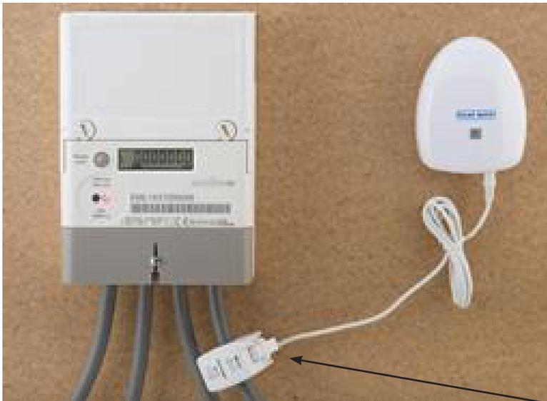
**IMPORTANT:** the orientation markings on the clamp must be observed to ensure only excess current is detected and used for water heating.
