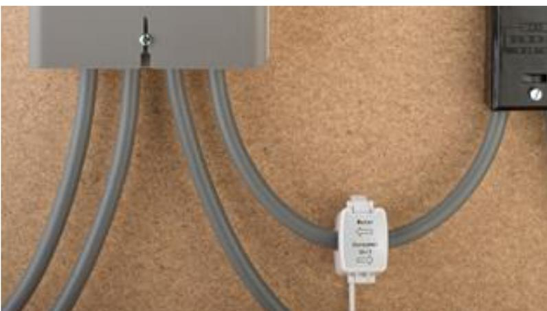
Henley or other connector block is fitted, the Measurement Clamp is fitted between the utility meter and the connection block.
