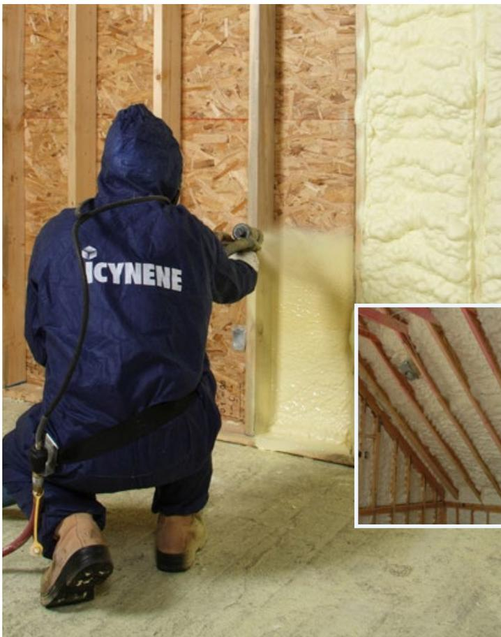
SPRAY FOAM INSULATION PROVIDES AIR SEALING, WHICH PREVENTS HEAT LOSS, SAVING YOU MONEY
